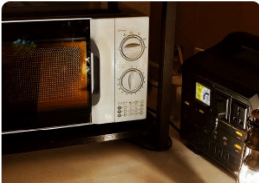
Backup Emergency Power
